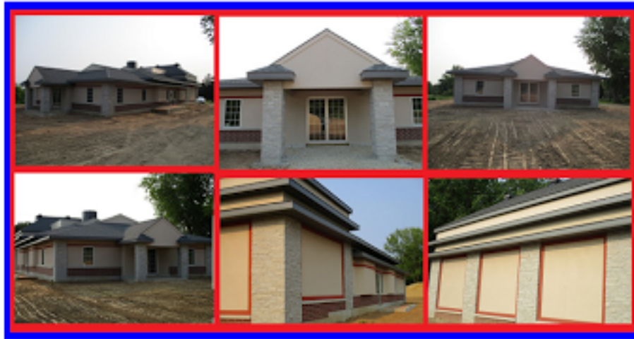
The Temple and Community Center Building: Main Structure Completed
